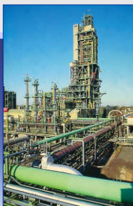
HTW pressurized gasification 1) 1986-1992 throughput 13 t/h 3)
